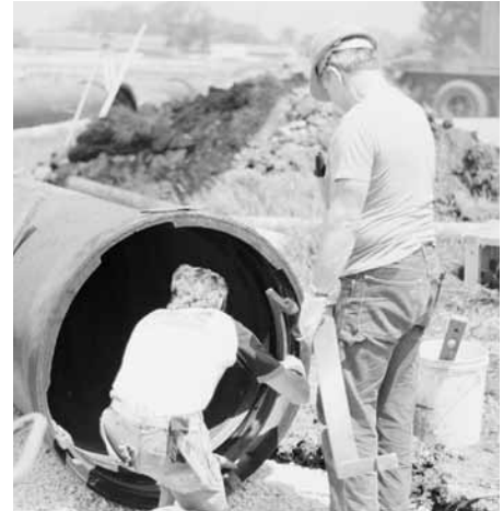
Figure 21: TR FLEX GRIPPER Ring Installation
