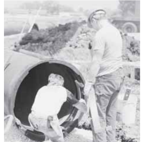
Figure 21: TR FLEX GRIPPER Ring Installation
